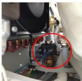
Normal-open Valve (Blue line)
