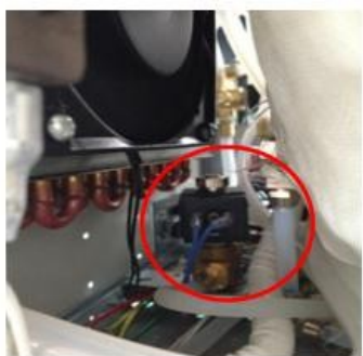
Normal-open Valve (Blue line)
