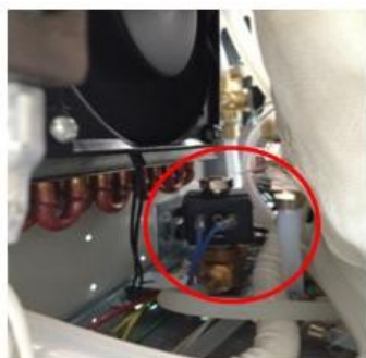
Normal-open Valve (Blue line)
